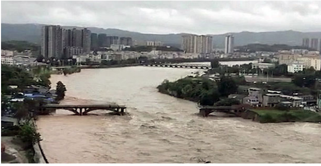
A bridge destroyed by floods in southwestern China's Sichuan province, July 2018.
